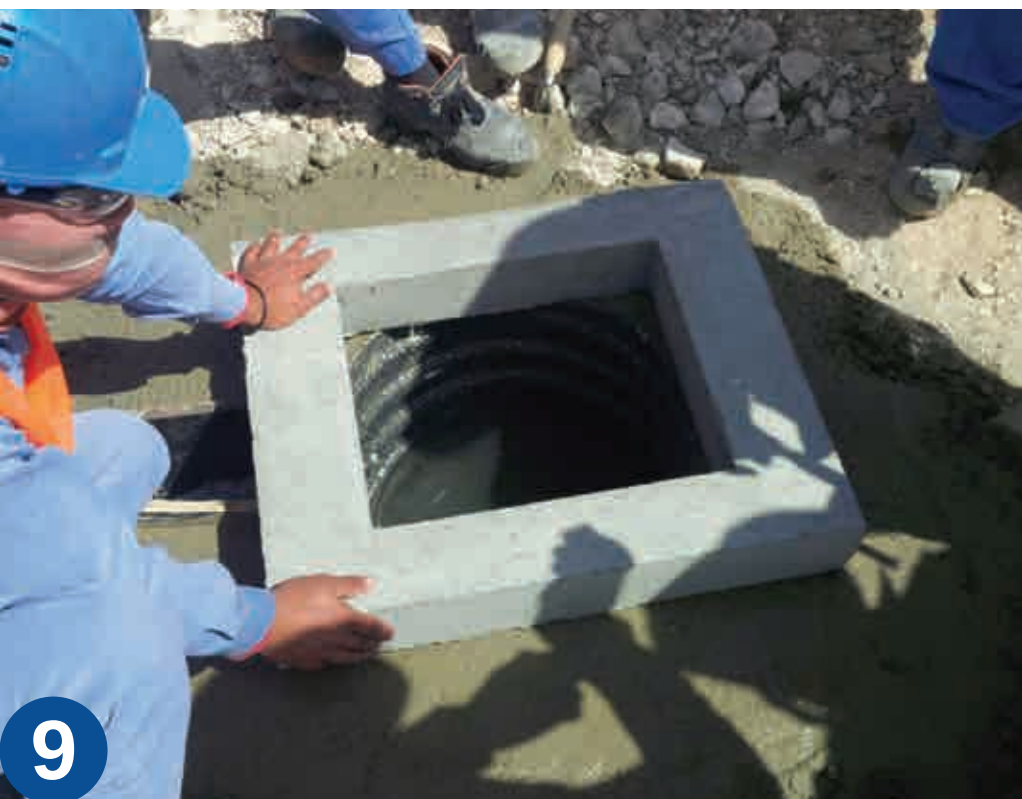
Place concrete pad on level surface
