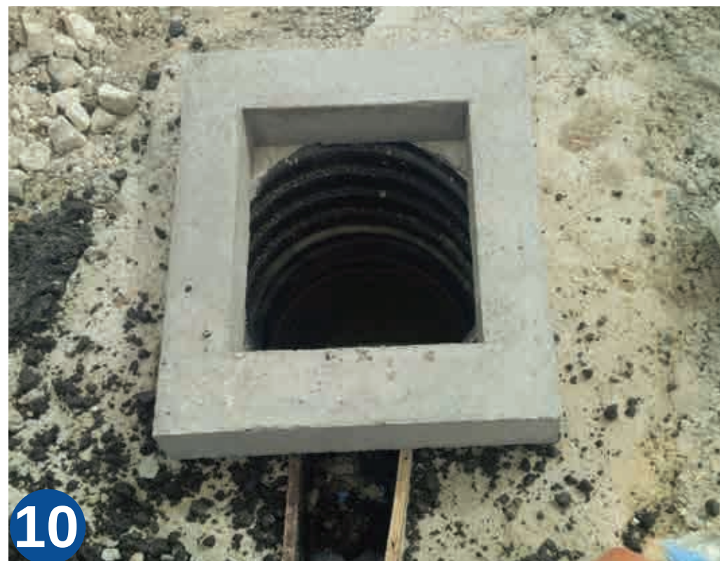
Finished install - Ready for gully grating & finished surface level
