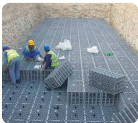
Polystorm installation
