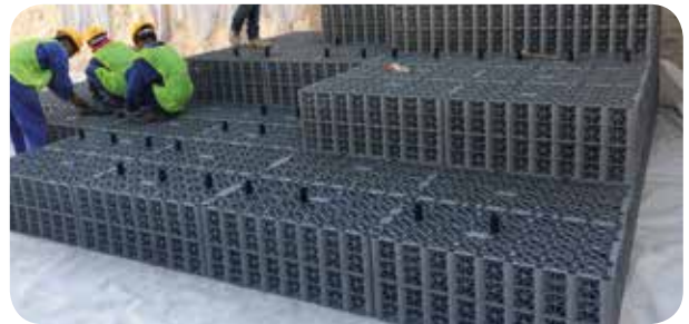
4 Always begin installation from corner to ensure correct alignment
