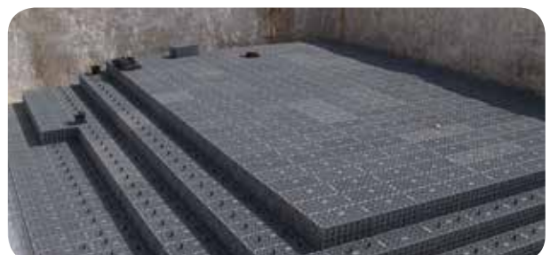
8 Typical speed of installation 400m³/day (team of 12)
