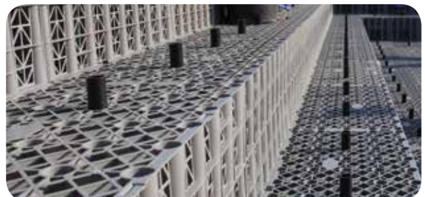
6 Lock polystorm units together utilising supplied shear connectors and 'U' clips
