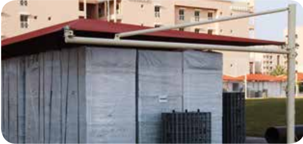
1 On-site storage (UV protection)
