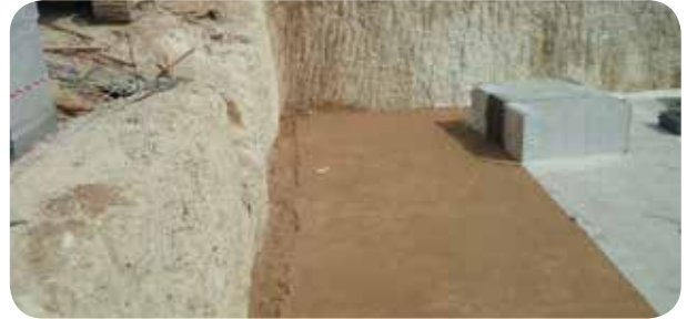
2 Excavation, base preparation and geotextile fabric
