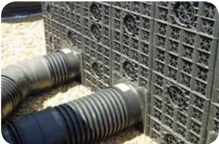
Polystorm cell with Drainage Flange Connection
